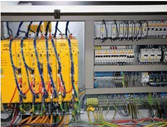
▲ Among other things, the control cabinet planned and produced by Baumüller has the control technology with the stackable servo inverter series b maXX 5000
